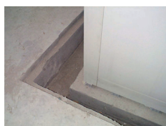
Excavation sample Dettaglio scavo
